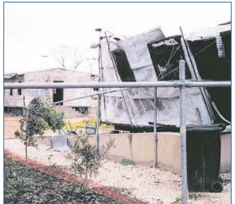
Burnt out dormitories at Port Hedland detention centre following riots
