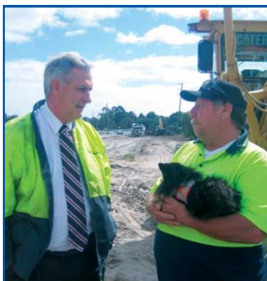
Barry Hahn and 'Little Man' show Mr Randall the progress being made along Ranford Road.
